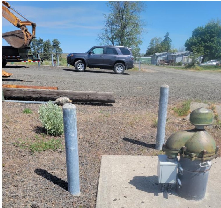
Figure 4 – South Well (Well #1) in Foreground, North Well (Well #2) in Background
